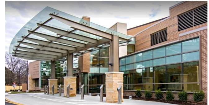
Women's Hospital Entrance at Henrico Doctors' Hospital
